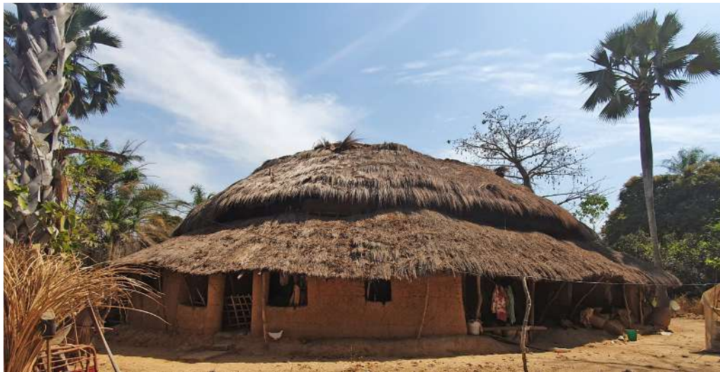
ENAMPORE IMPLUVIUM HUT 1: Front view, 2, 3, 4: Views from the inner courtyard
